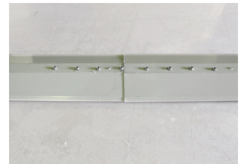
Finished Spliced Ridge Beam
